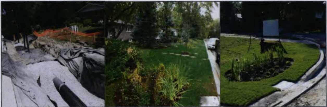
Forest Glen project construction and LID features (Photo credit: LSRCA)
