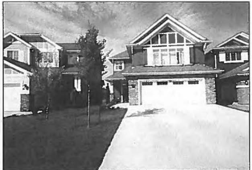
Figure 2: Visitable home with a no-step level entrance beside a home with steps leading to the front door Photo by Ron Wickman
