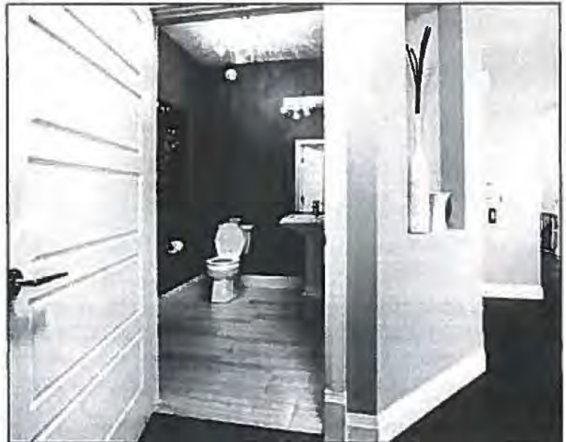
Figure 11: A toilet with sufficient transfer space adjacent Photo by Ron Wickman
