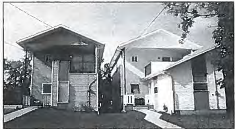
Figure 4: Visitable home, on left, with sloping sidewalk and no-step entrance located at the back of home Photo by Ron Wickman
