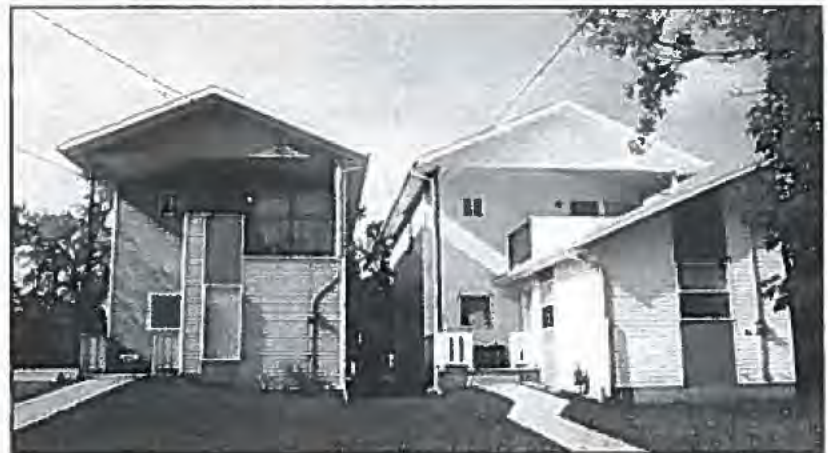
Figure 4: Visitable home, on left, with sloping sidewalk and no-step entrance located at the back of home Photo by Ron Wickman
