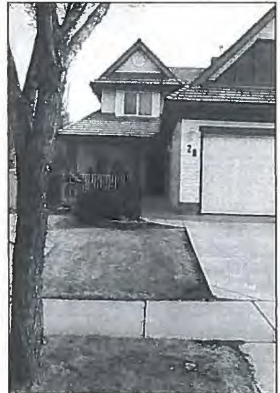
Figure 1: Visitable home complete with a no-step front entrance Photo by Ron Wickman
