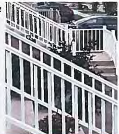
New Oshawa streets have houses with 8, 9, even up to 15 steps to the front door.
