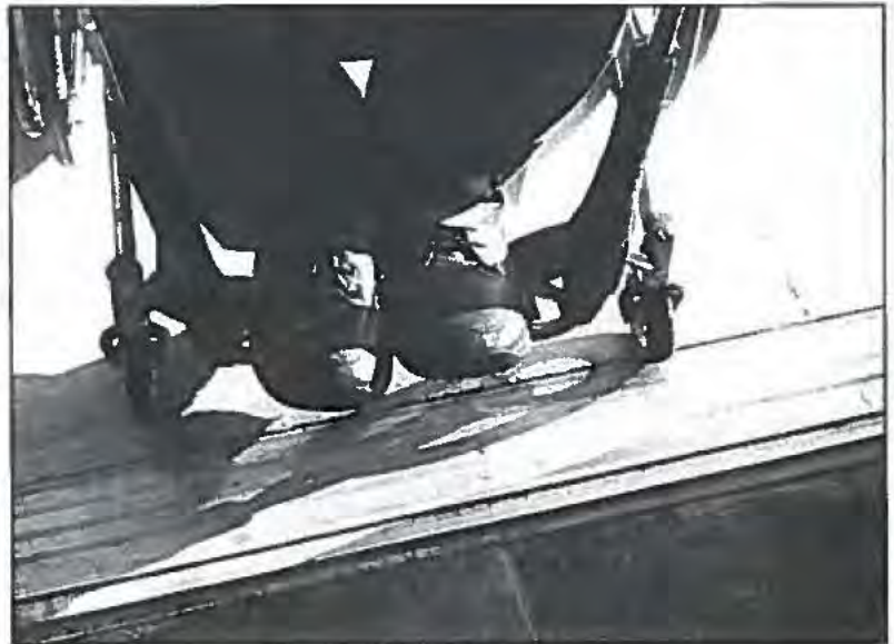
Figure 9: Low profile door threshold Photo by Ron Wickman
