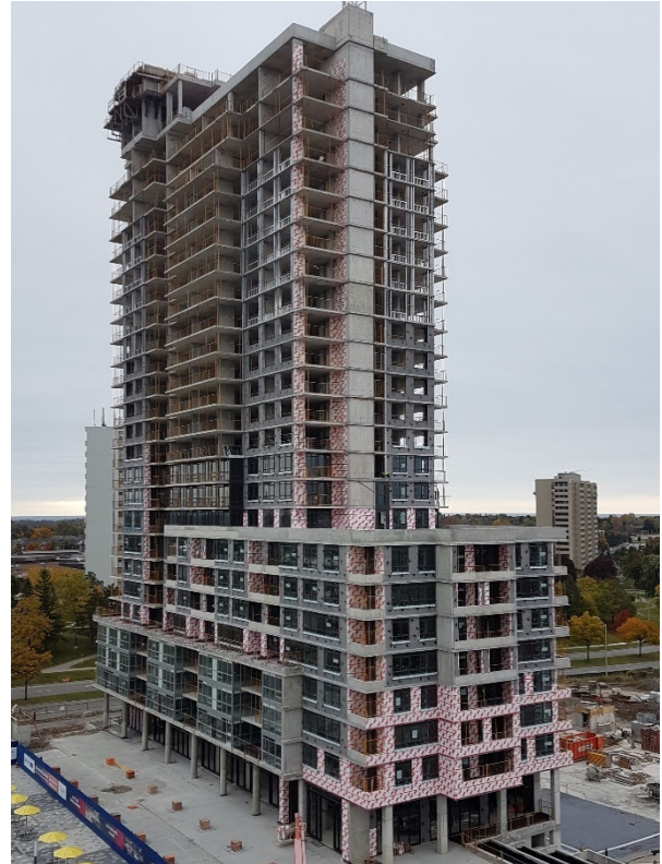
Figure 27: Market rental apartments under construction at Vision at Pat Bayly Square in Ajax, a project that received funding and support through Ajax's Downtown CIP program, the Regional Revitalization Program and CMHC.
