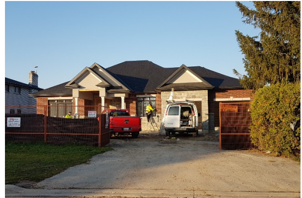
Figure 20: An example of a single-detached home which was demolished and rebuilt.
