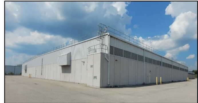
NSS-D Used Fuel Dry Storage Building (UFDSB) #2
