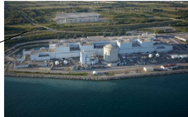
Darlington Nuclear Generating Station
