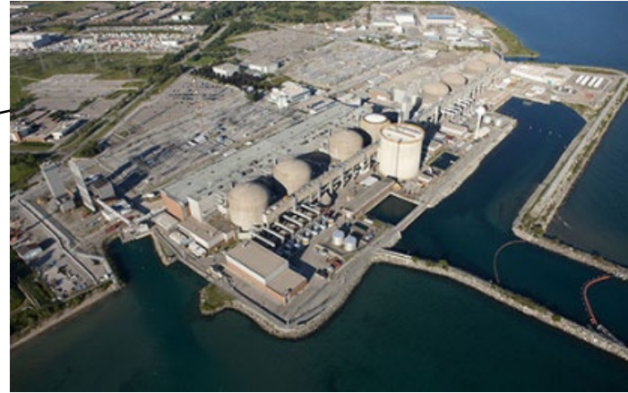
Pickering Nuclear Generating Station
