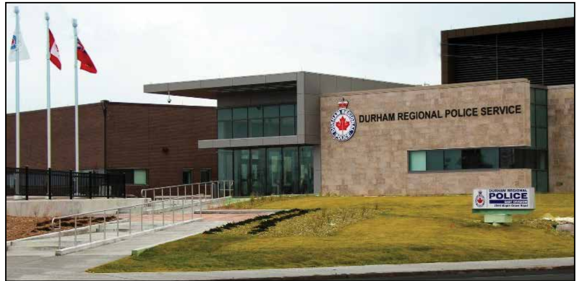
New Clarington Police Complex
