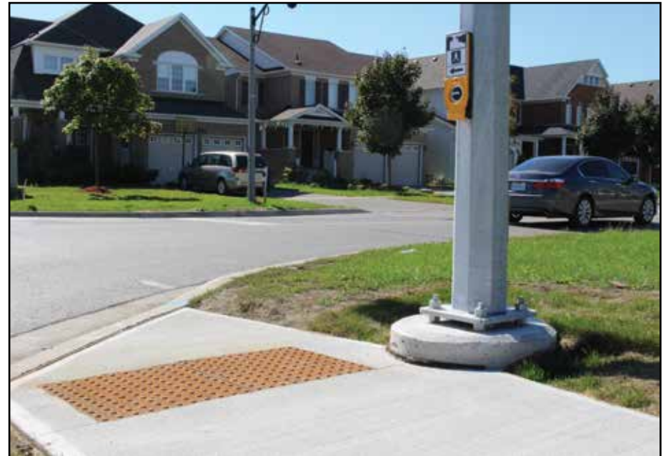
Example of an intersection with an APS and tactile walking surface indicator
