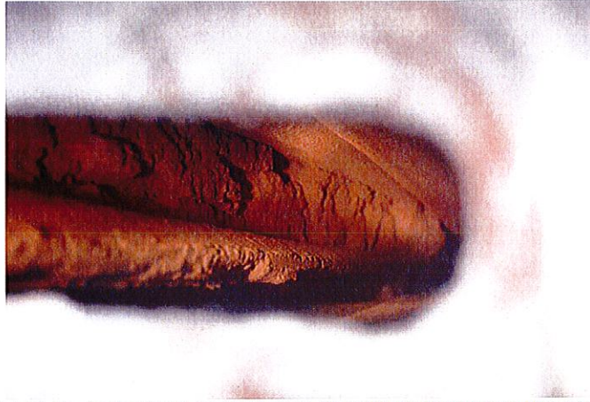
Photo 24 - View Looking Through Hole in Tubesheet - Shows Plugging Between Bags - NOT TYPICAL
