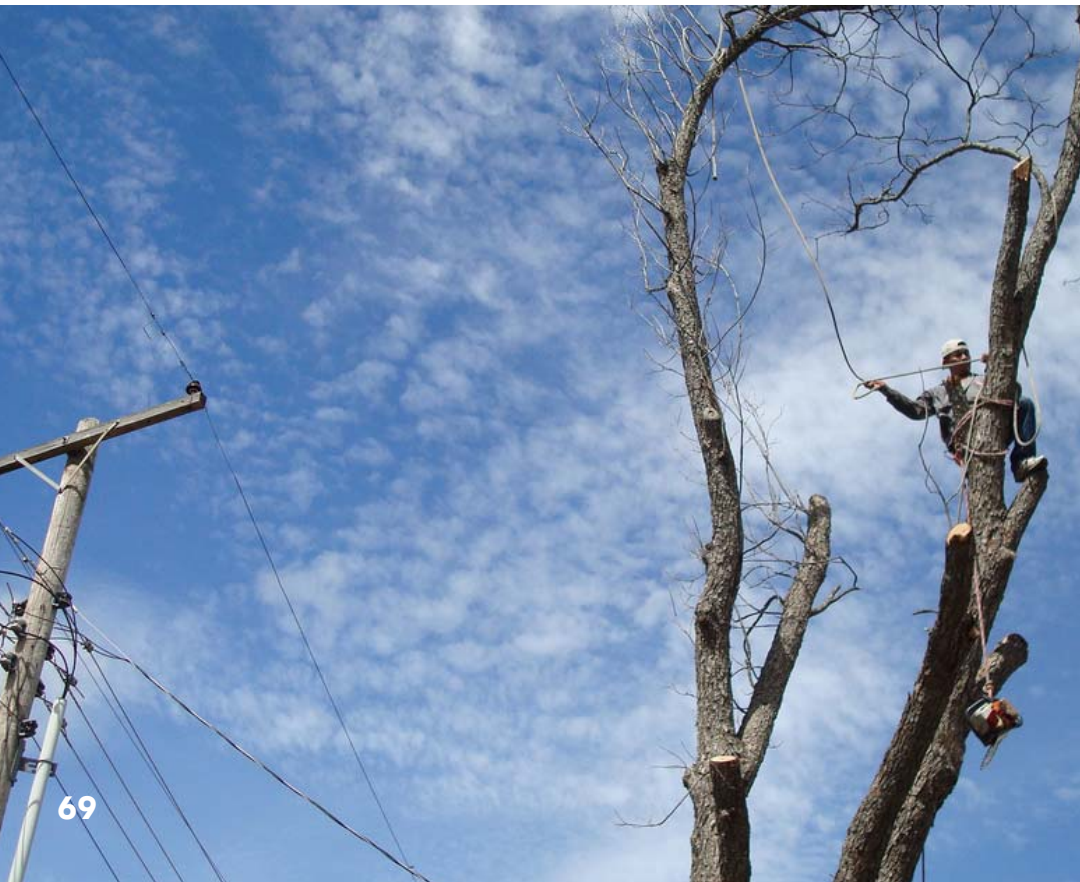
◀ An arborist trims tree limbs away from electrical lines
