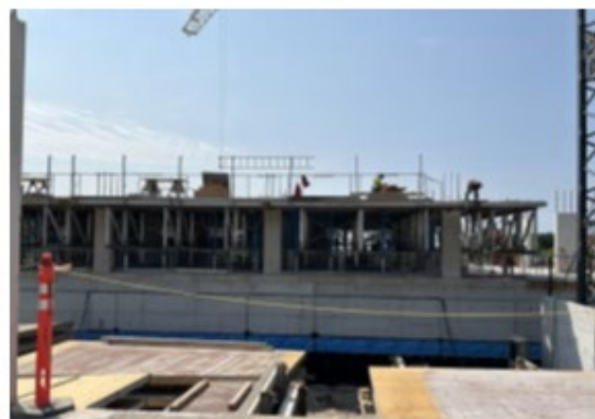
Current Site View
