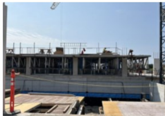
Current Site View
